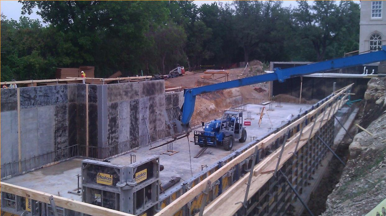
This is a progress photo of the cistern installation. This photo shows the immense scale of the cistern, which measures 26' wide x 132' long x 14' tall with 12" thick reinforced concrete walls. You will notice how small the all-terrain forklift appears as it is parked in the middle of the cistern. This photo also shows how strict safety measures were adhered to including the safety scaffolding and shoring in place.
