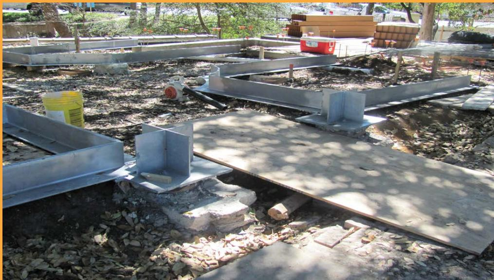
An engineered pier-and-beam construction technique minimized the impact of the hardscape on the existing tree. Fabricated steel beams reduced the number of piers needed. The seat walls were built on the steel beams to allow them to “float” above the root system of the existing tree.
