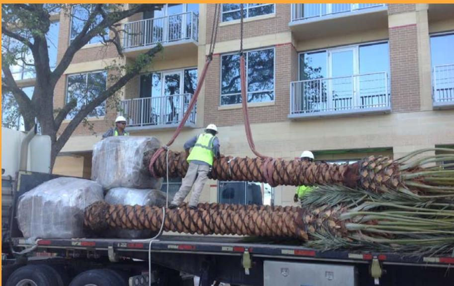
All materials were crane lifted; 610 lifts in total. Each of the trees was rigged to balance the palms in an upright position to plant directly into the roof-top planters.
