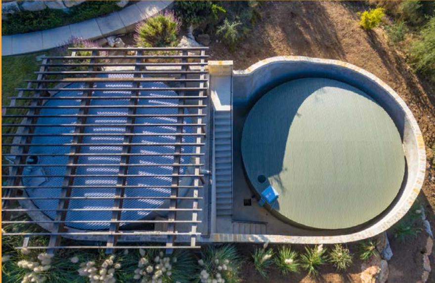
Three fourths of the upper tank was placed below grade. The masonry walls provide slope retention and act as a visual barrier to the tank. To further screen the view an arbor was designed and built on top to reduce the visual impact from surrounding properties.
