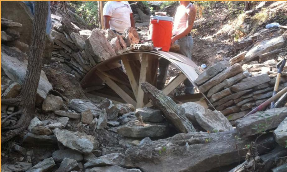
Natural looking and remotely located with limited access, no electricity, and able to withstand heavy torrents of water at times; the only logical solution was to go old school. The Romans have the best solutions. A dry stacked arch bridge was the best way to achieve the goal considering the list of challenges.
