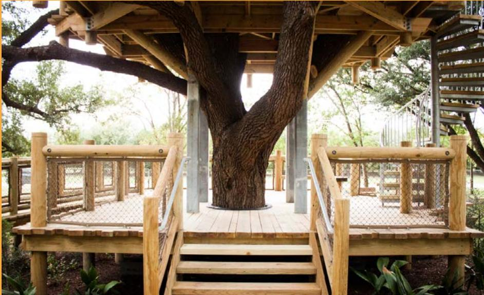
Formal entrance to treehouse from atop levee. Only one branch was removed to allow for construction (upper right.) Nowhere did we attach directly to tree. Full-thickness lumber used at treehouse decking for increased strength across larger spans. (Note crenelated equal board lengths at approach below.)
